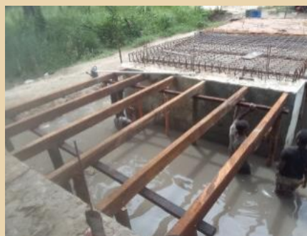
Bridge structure ©GNAP
