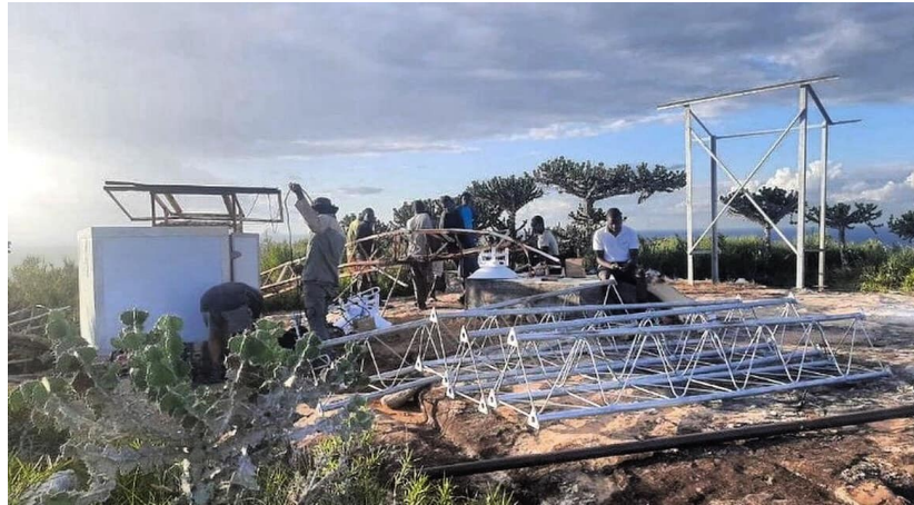
Setting up the radio system ©GNAP
