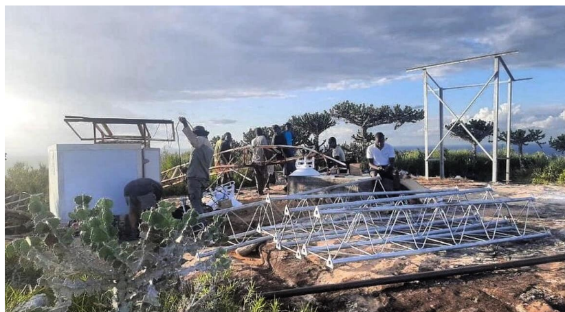
Antenna's system installation ©FFS-IGF
