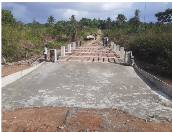
Rehabilitation of the Mulela bridge ©GNAP
