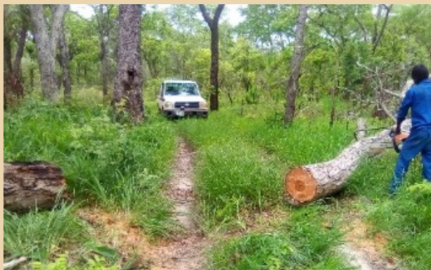
Road maintenance ©GNAP
