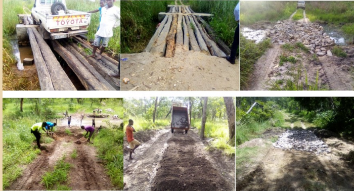
Roads and bridges maintenance ©GNAP
