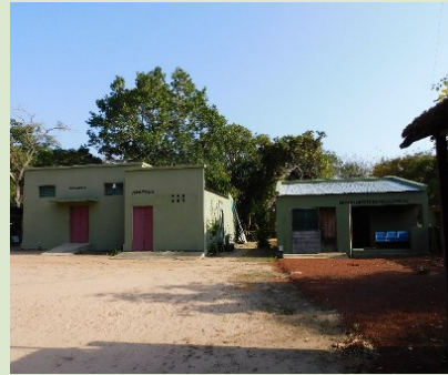
One of the staff accommodation and the warehouse ©GNAP
